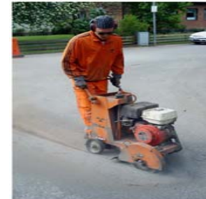
Figure 4: Micro trenching on the pavement
