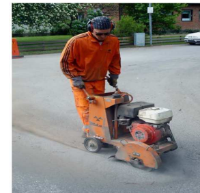
Figure 4: Micro trenching on the pavement
