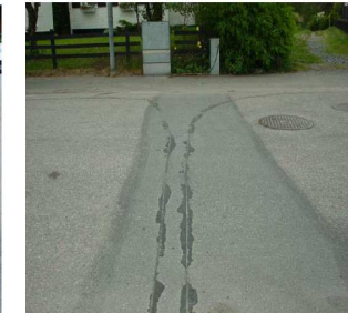
Figure 5: Fiber grooves on the pavement
